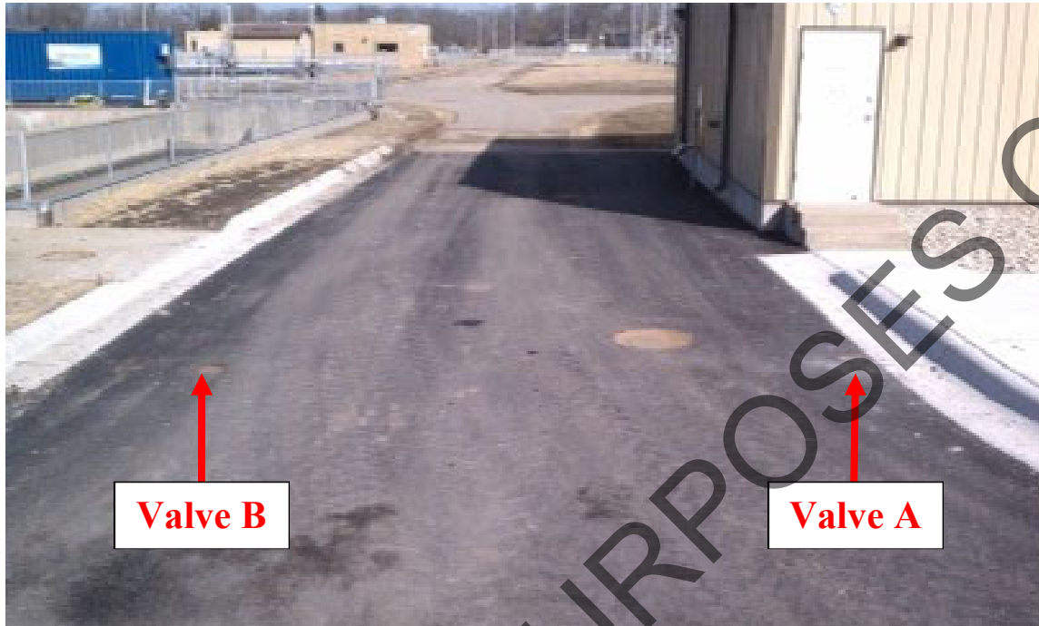
FIGURE 1: Spill Containment Valve Locations
