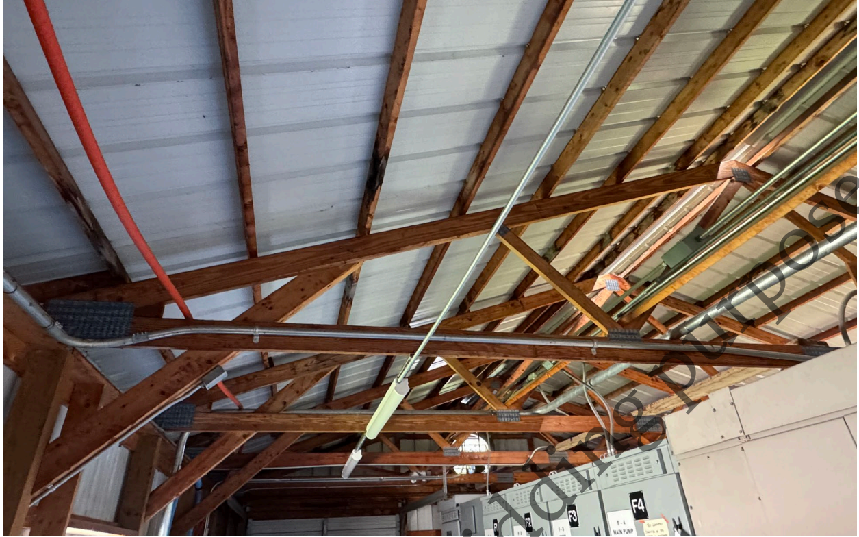
Switchgear Building Rafter and Purlin Substructure
