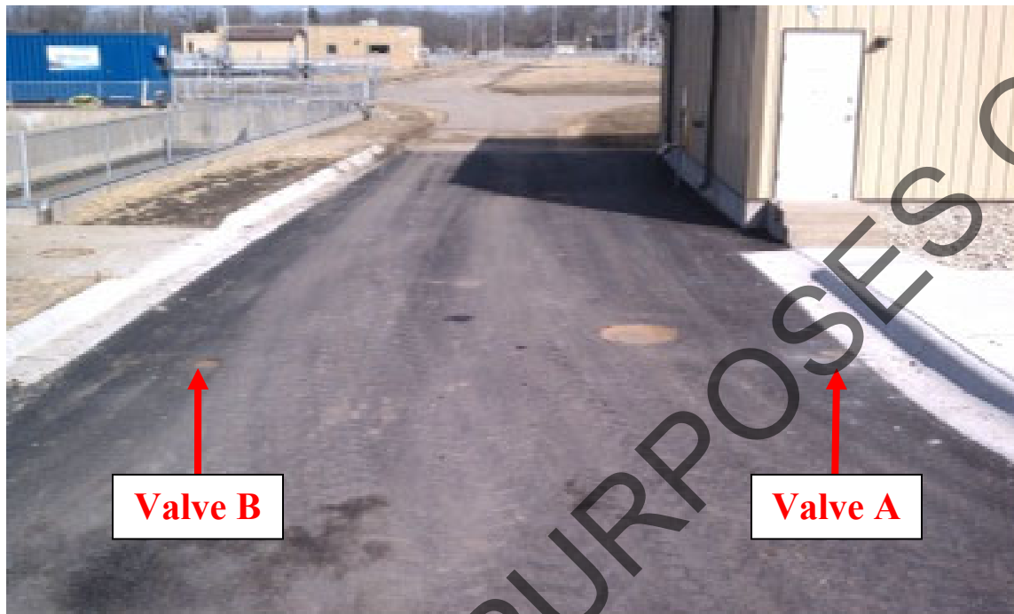
FIGURE 1: Spill Containment Valve Locations
