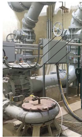
PUMP NO. 2 TERMINAL BOX
