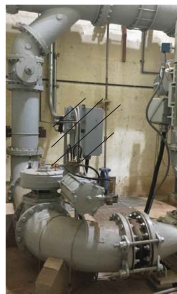
PUMP NO. 3 TERMINAL BOX
