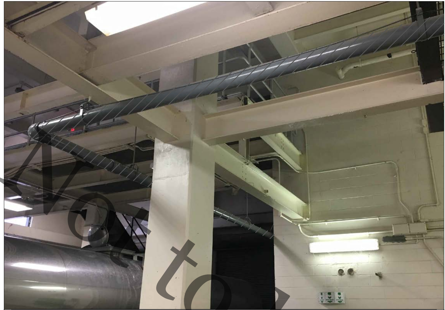
2 4" POLYMER SUPPLY 3 SCALE: NONE
