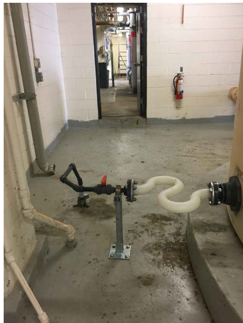
10 EX. TANK OUTLET PIPING 3, 5 SCALE: NONE
