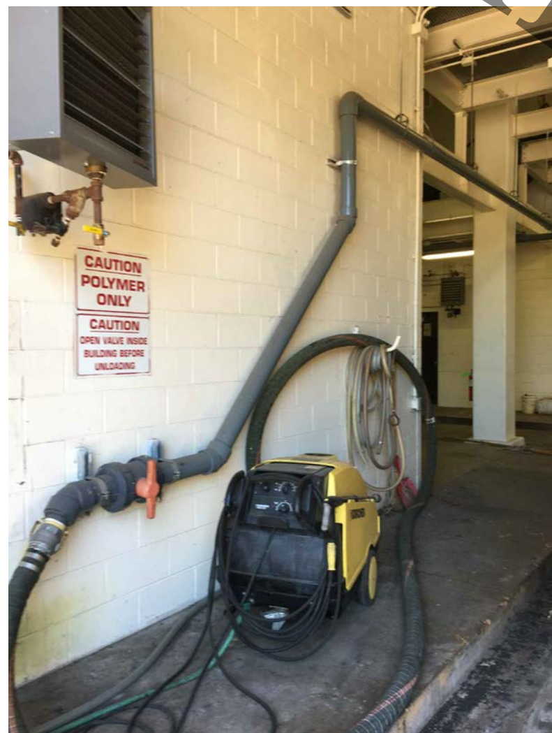
11 EX. 4" PVC POLYMER FILL LINE 5 SCALE: NONE
