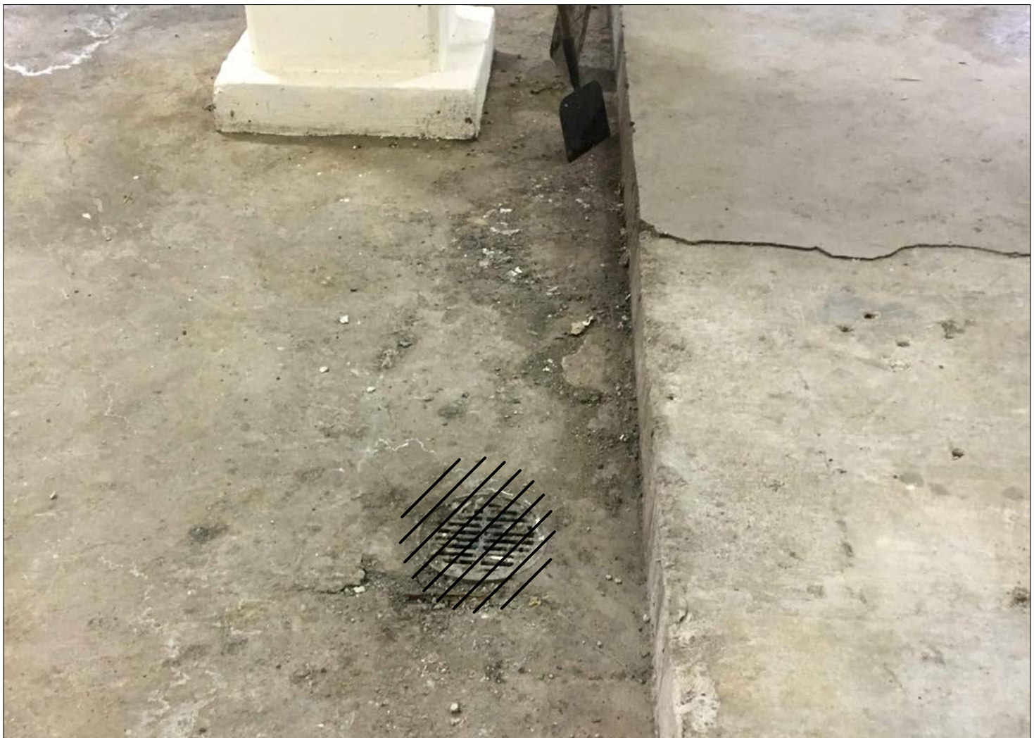
7 FLOOR DRAIN TO BE REMOVED 3 SCALE: NONE
