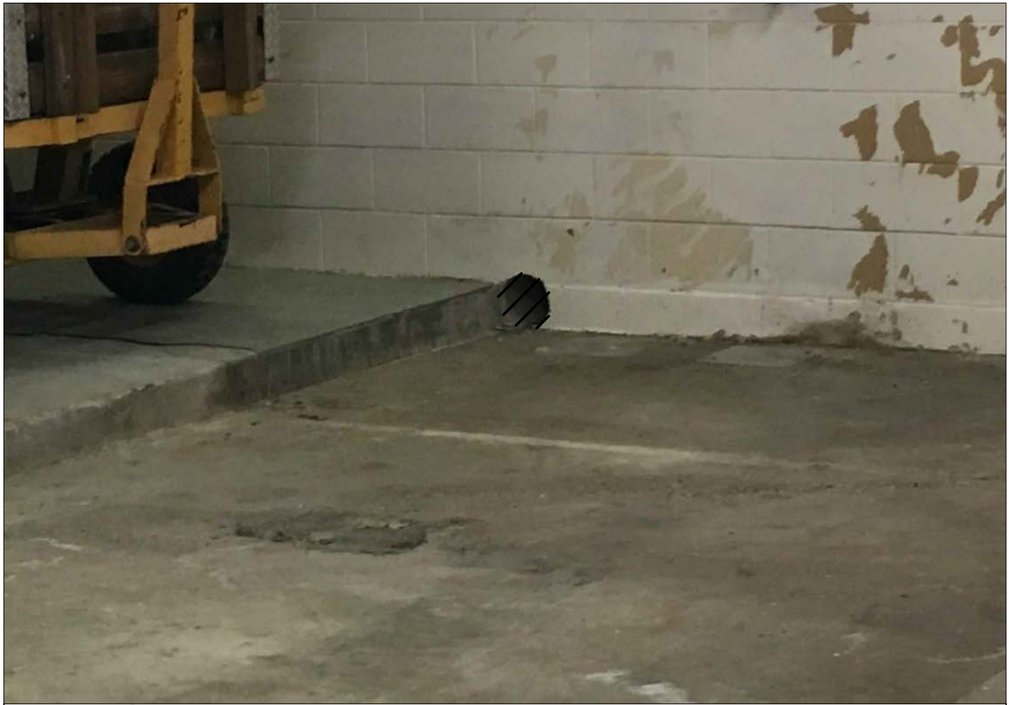
3 6" HOLE IN WEST WALL TO BE PLUGGED 3 SCALE: NONE
