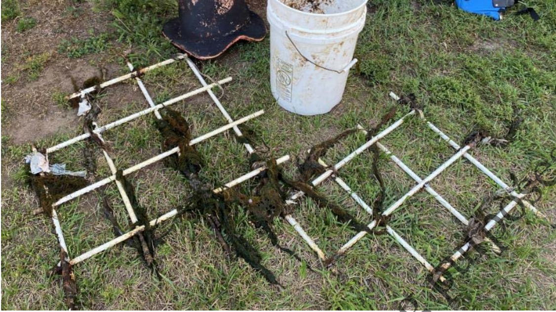
Figure 5: Removed Sections of Existing Debris Screen
